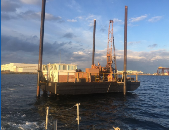
SELF-ELEVATING BARGE OR 'LIFTBOAT'
