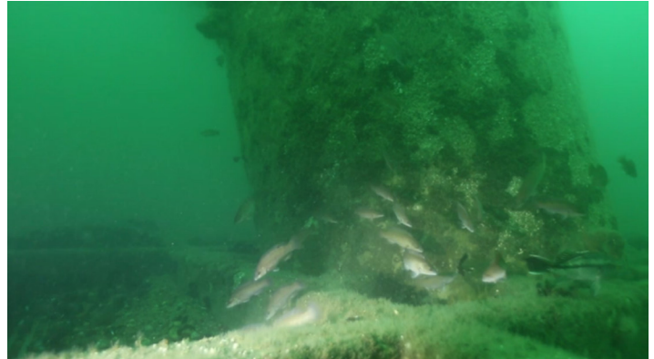
↑ The foundations at Block Island Wind Farm, acting as an artificial reef.
