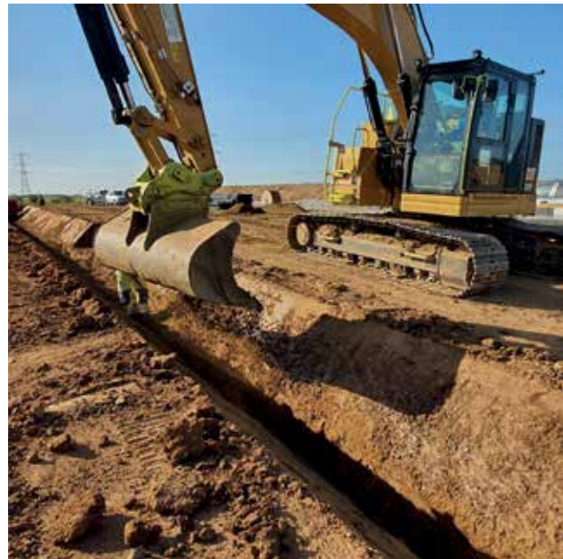
Onshore construction activities along the cable route
