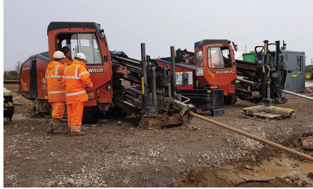
Horizontal Directional Drilling underway along the cable route.
