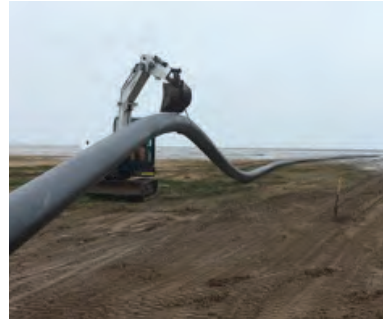
Duct pre installation in the intertidal area
