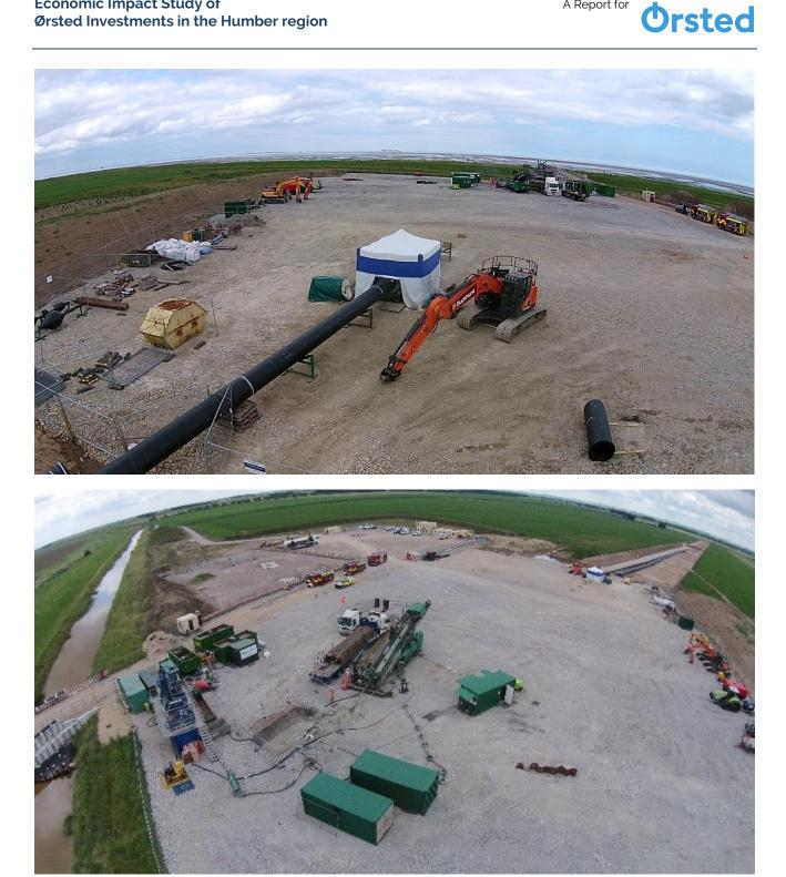
Figure 8 - Hornsea 2 cables being pulled through for onshore connections
