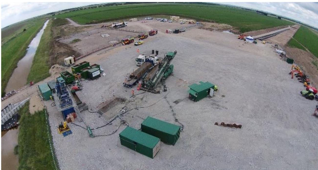
Figure 8 - Hornsea 2 cables being pulled through for onshore connections
