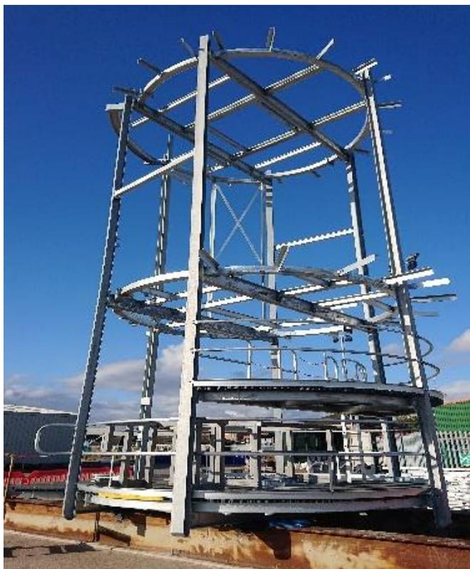
**Figure 10 - Internal platform structures for Hornsea 2's offshore wind transition pieces**
