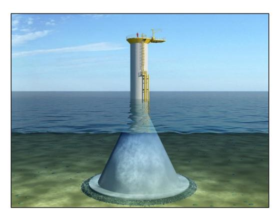
Figure 3.5 A gravity base foundation.
