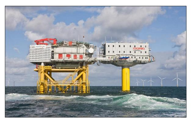
Figure 3.8 Offshore accommodation platform (right) at the Horns Rev 2 offshore wind farm, sited next to an offshore substation (left)\*.
