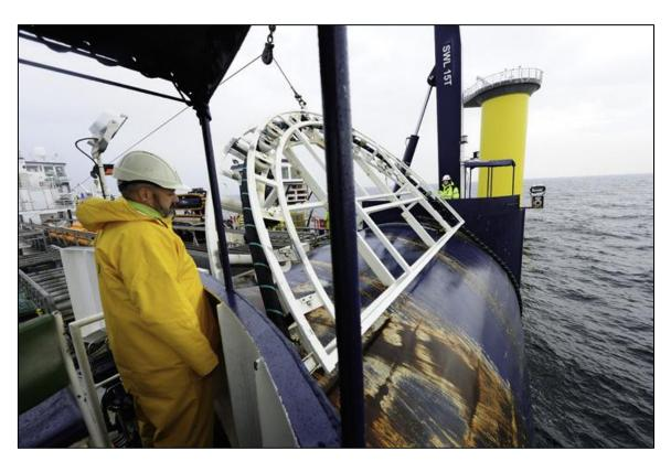
Figure 3.7 Array cable installation at the Gode Wind offshore wind farm.
