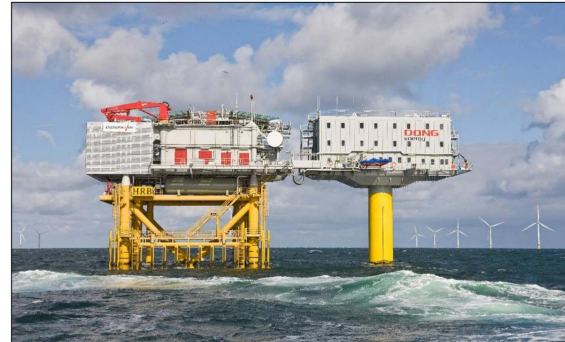
Figure 3.13: Offshore accommodation platform (right) at the Horns Rev 2 offshore wind farm, sited next to an offshore substation (left)<sup>2</sup>.
