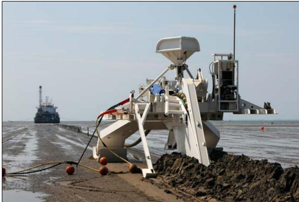
Figure 3.20: Example of a cable plough pulled from an installation vessel. (Source: <http://www.4coffshore.com/s/about/equipmentTypes.aspx>)
