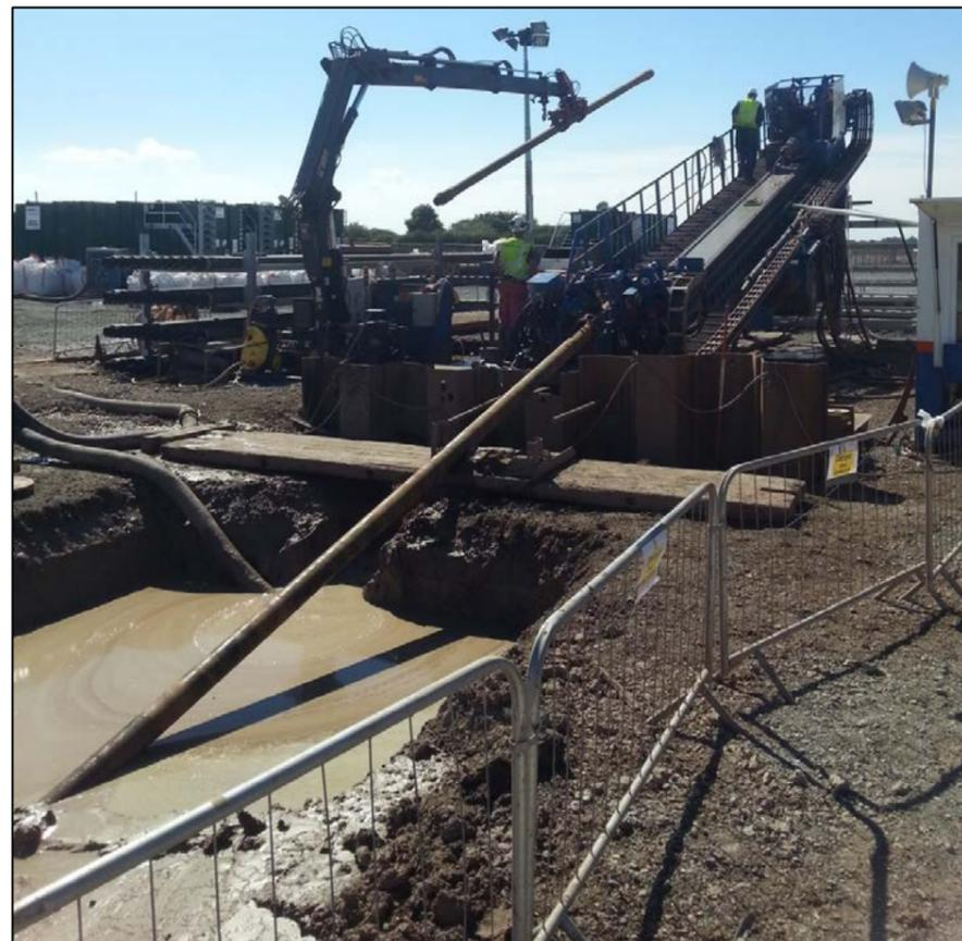
Figure 3.19: HDD rig carrying out landfall works at the Westermost Rough Offshore Wind farm.
