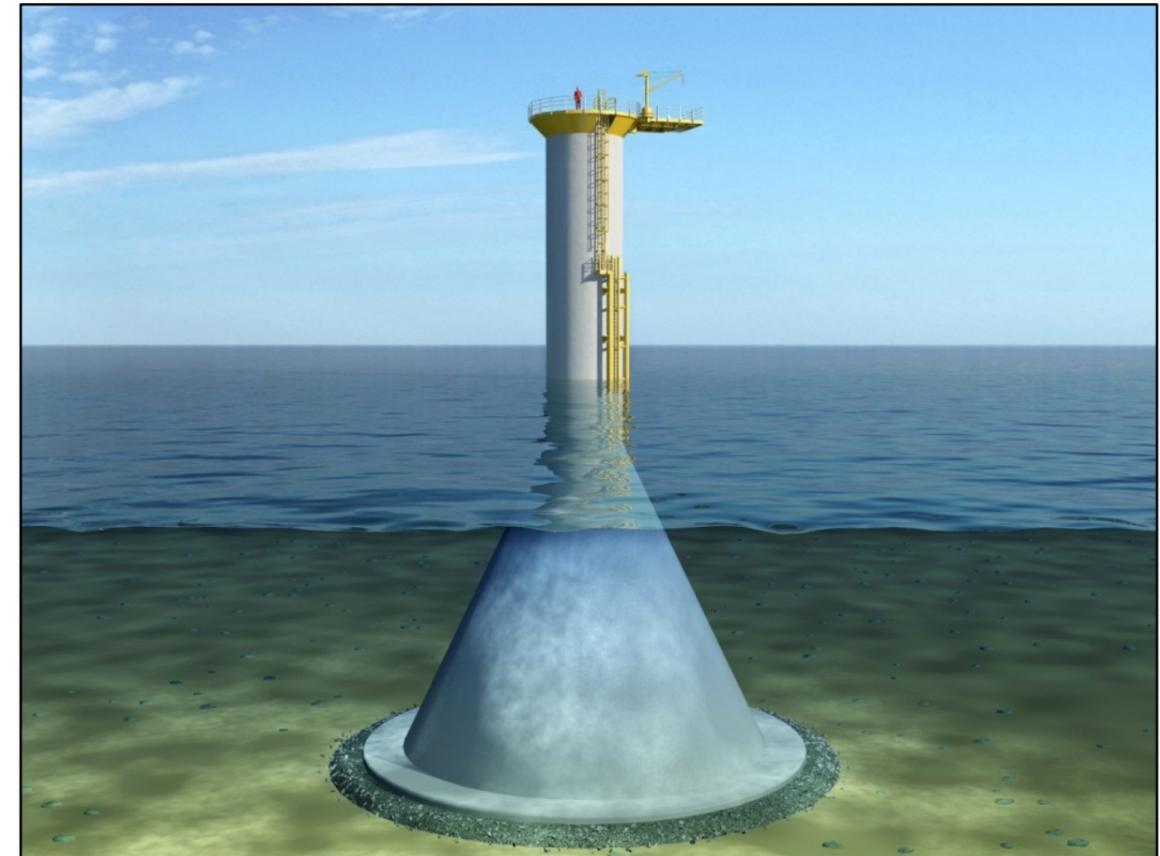
Figure 3.9: A gravity base foundation.
