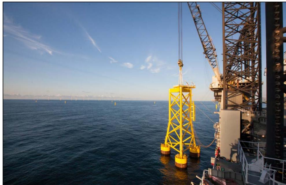
Figure 3.8: A jacket foundation with suction buckets being installed at the Borkum Riffgrund One offshore wind farm.
