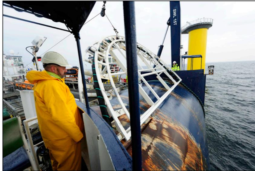
Figure 3.12: Array cable installation at the Gode Wind offshore wind farm.
