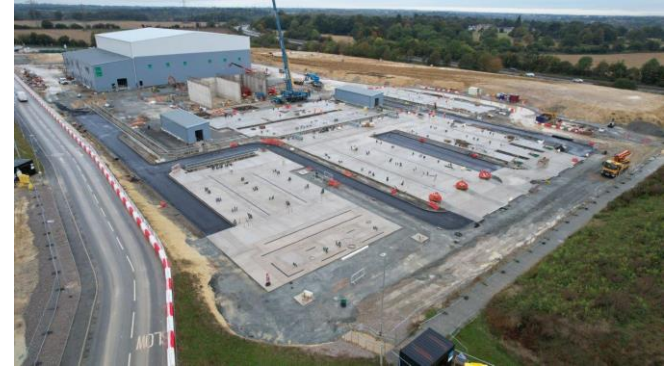
AC yard, cable pits and duct installation
