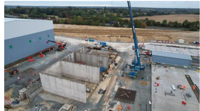
Transformer bays and relay building
