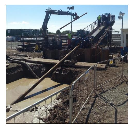
Figure 3.23: HDD rig carrying out landfall works at the Westermost Rough offshore wind farm.
