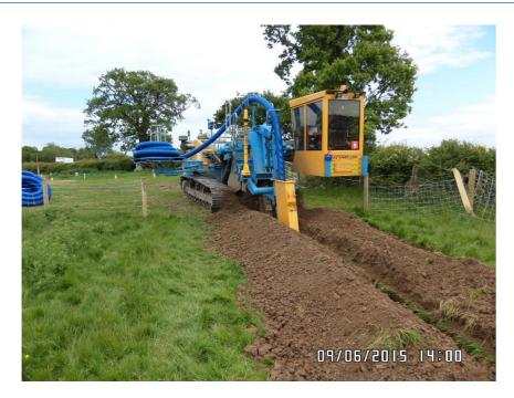
Figure 3.26: An example of a tracked tool used for pre-construction drainage.
