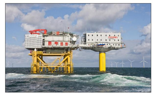
Figure 3.16: Offshore accommodation platform (right) at the Horns Rev 2 offshore wind farm, sited next to an offshore substation (left)<sup>2</sup>.
