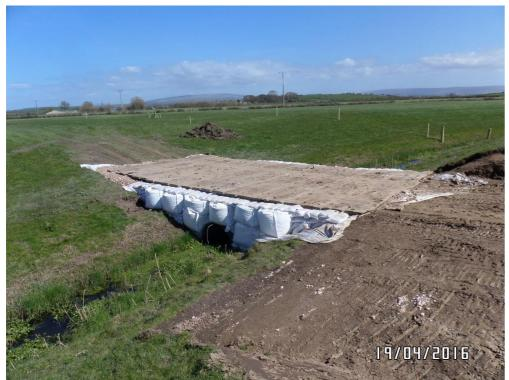
Figure 3.28: A sample flume installation.
