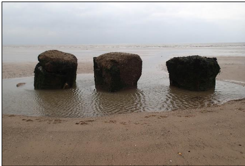
Figure 32: Example of scour around rank traps (IECS, 2019).
