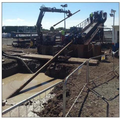
Figure 4.15: HDD rig carrying out landfall works at the Westermost Rough offshore wind farm
