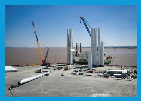
Wind turbine load-out to DEME's Sea Challenger in Hull. We have had two jack-up installation vessels working on the Wind Turbine Generator (WTG) installation campaign: DEME's Sea Challenger and Sea Installer. Both can carry four full WTG sets each, comprising three blades, one full tower section and a nacelle. It is hard to appreciate the scale of this enormous vessel, but when you remember that each tower is roughly the height of Grimsby's dock tower, it puts the scene into perspective!
