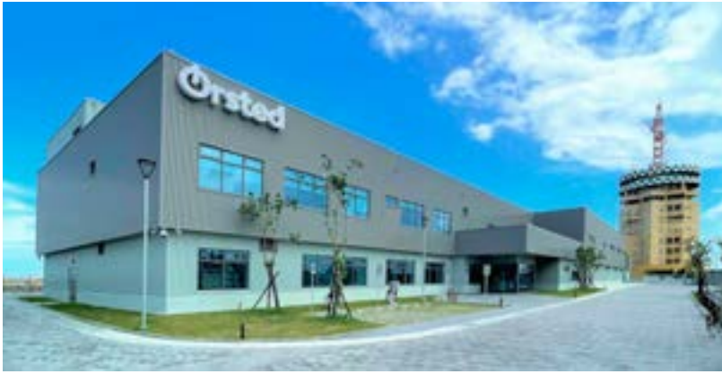
⤴ Ørsted Taiwan Offshore Wind Farm Operation and Maintenance Hub at the Port of Taichung
