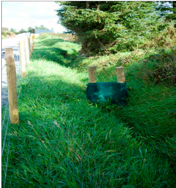
Figure 2-1: Silt Trap across Grassed Swale
