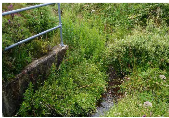
Plate 1.7: Drainage Ditches (FW4)
