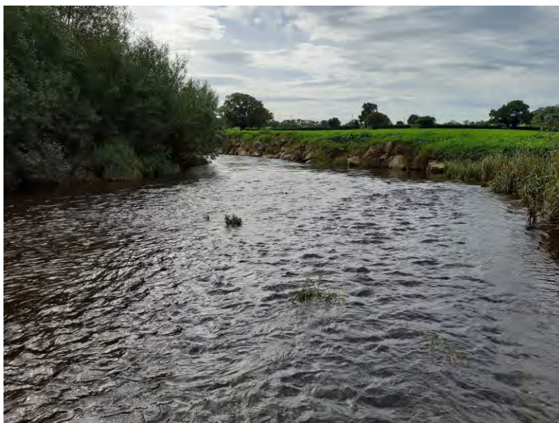
Photo 8: Clyda River. Bank Reinforcement
