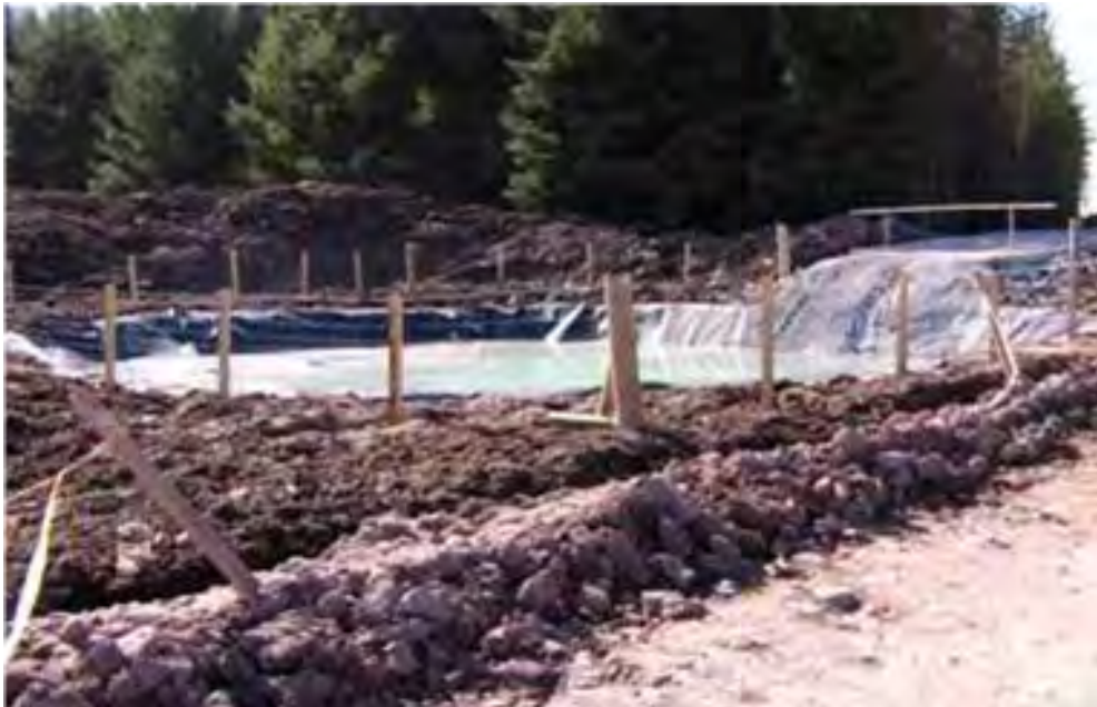
Figure 8: Lined Settlement Lagoon for Concrete Washout Facility
