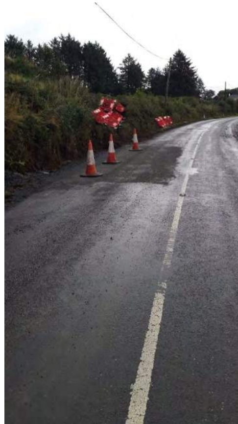
Plate 3-2: Typical Installation and Temporary Reinstatement of Joint Bay
