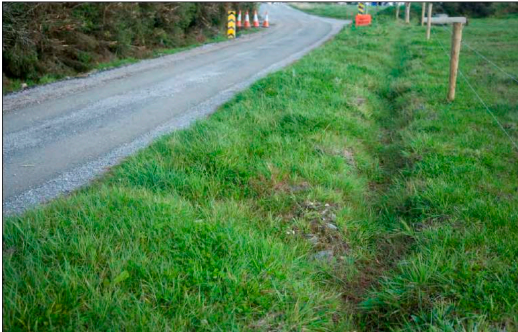
Figure 1: Grassed Swale along access track
