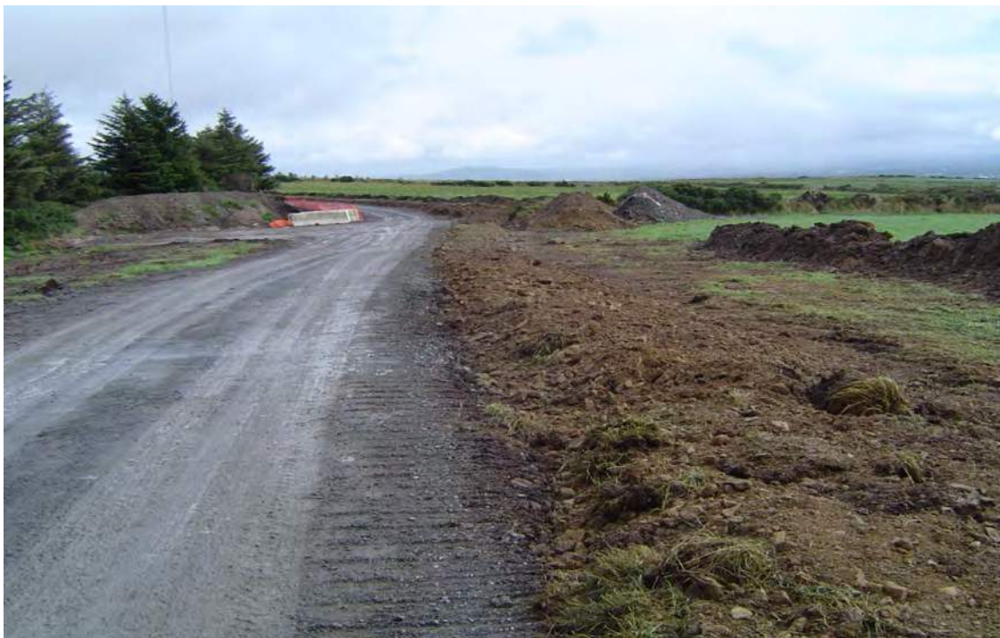
Figure 7: Backfill over Cable Trench
