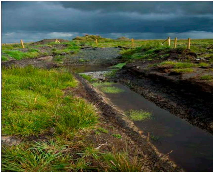
Figure 2: Swale draining to Settlement pond
