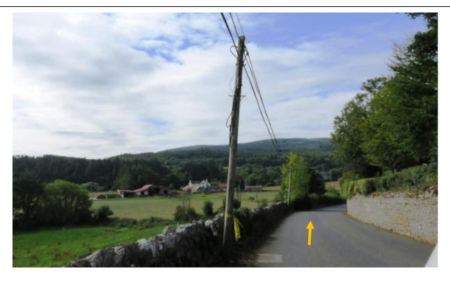
**Node 2.7.**A section of wall should be lowered to road level for mid oversail. Depending on rear overhang some load bearing may be required
