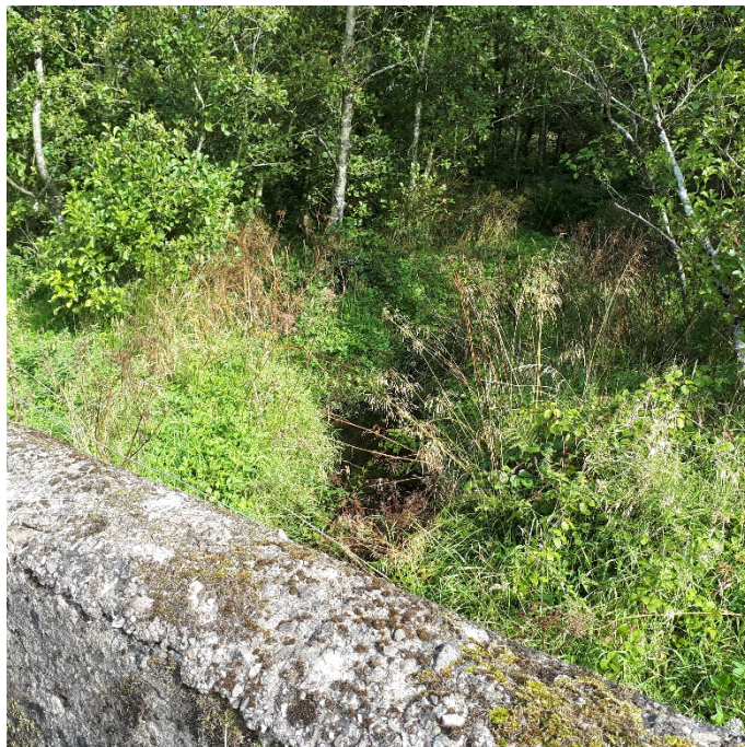
Viewpoint from the culvert looking upstream
