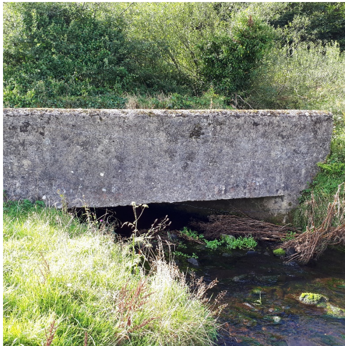
Viewpoint of looking upstream towards the culvert
