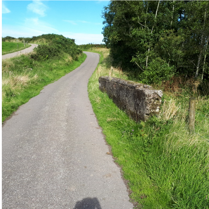
Viewpoint on the culvert
