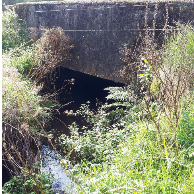
Viewpoint of looking upstream towards the culvert
