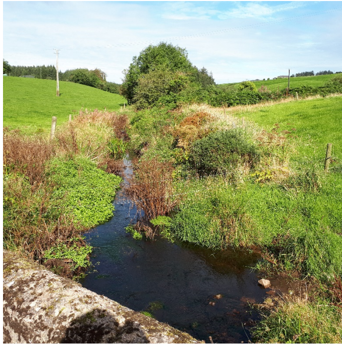
Viewpoint from the culvert upstream
