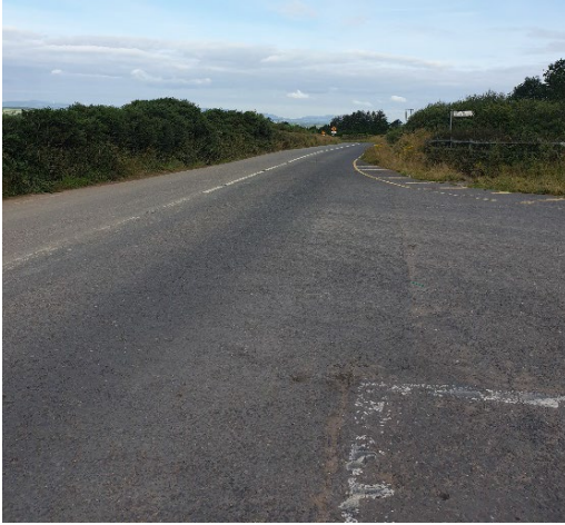
Plate 13-2: View Right from Bottlehill Landfill Site Entrance
