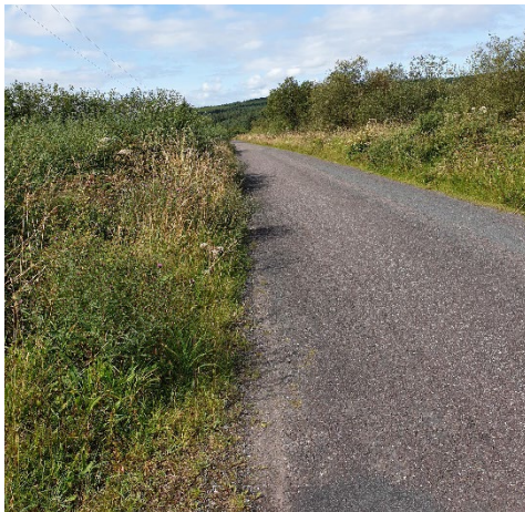
Plate 13-7: View Left from Lackendarragh Site Entrance
