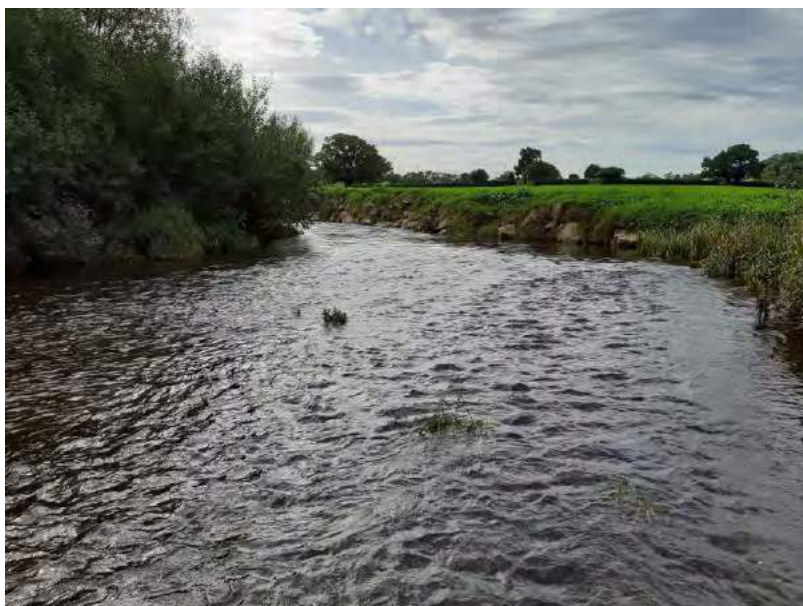
Photo 8: Clyda River. Bank Reinforcement
