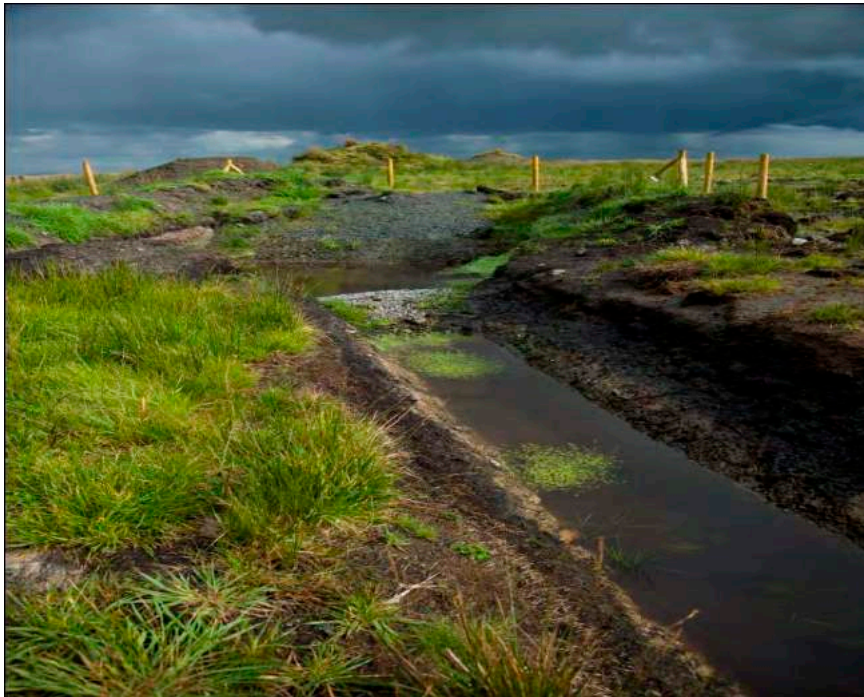
Figure 2: Swale draining to Settlement pond
