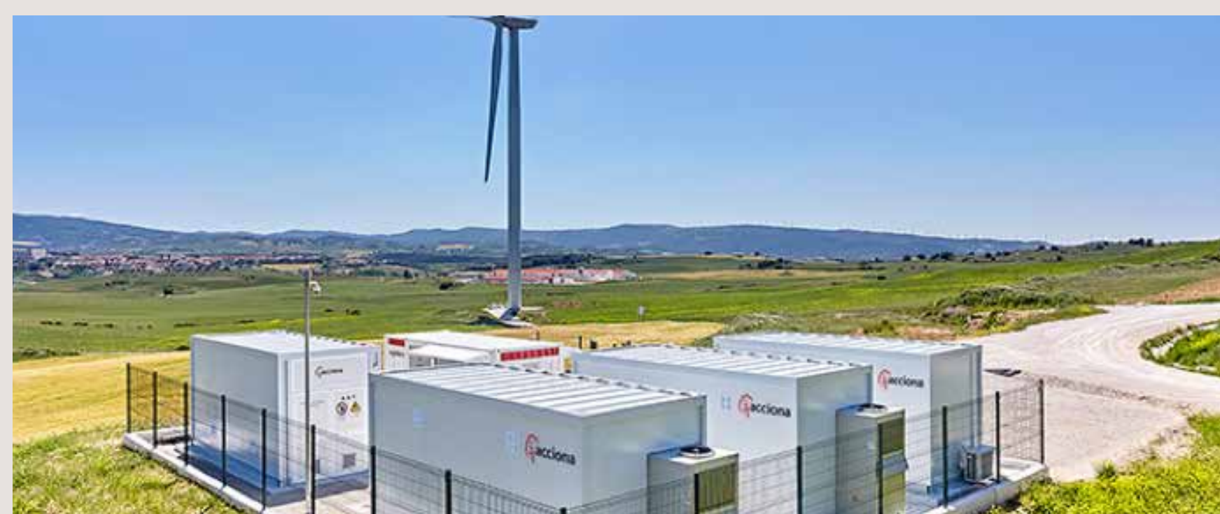
Hybrid plant for storing electricity in batteries that is part of a grid-connected wind farm in Spain
