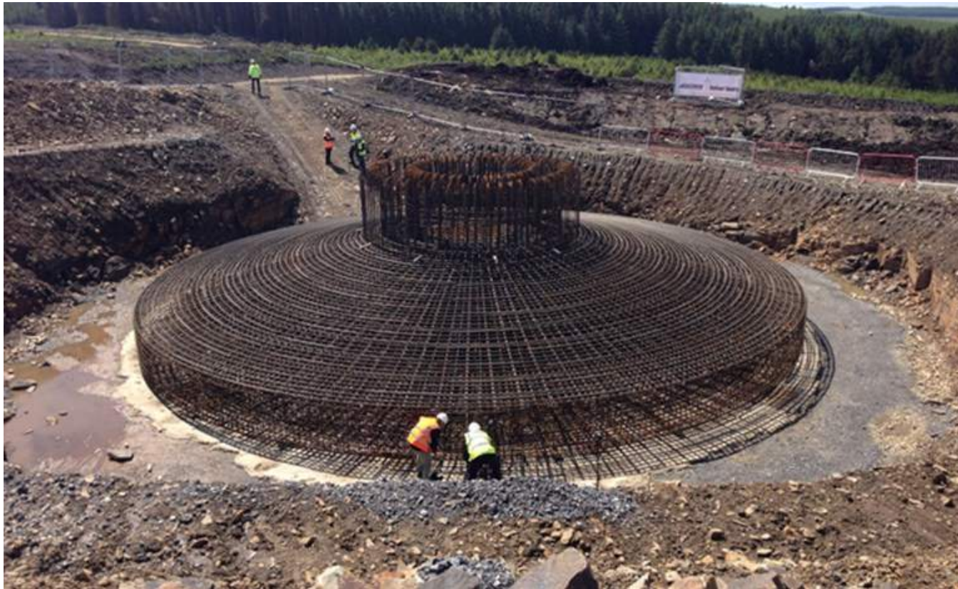
Turbine foundation reinforcement
