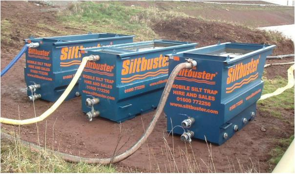
Figure 1-3 Temporary site settlement tanks (Source: Siltbuster)
