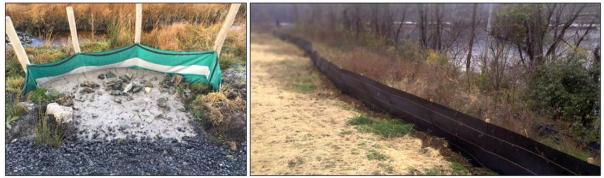
Figure 1-2 Silt fencing measures (Source: SSI Environmental (left) and Thrace Group (right)
