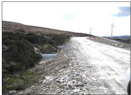
Figure 1-4 Typical example of stones used in a check dam to slow down water flow (Source: SNH, 2015)<sup>1</sup>
