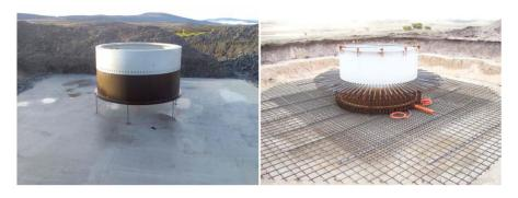
Plate 2-2: Levelled turbine tower "can" Plate 2-3: Steel reinforcement being added
