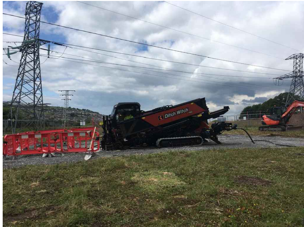
Image 1 : Typical Directional Drilling Rig
