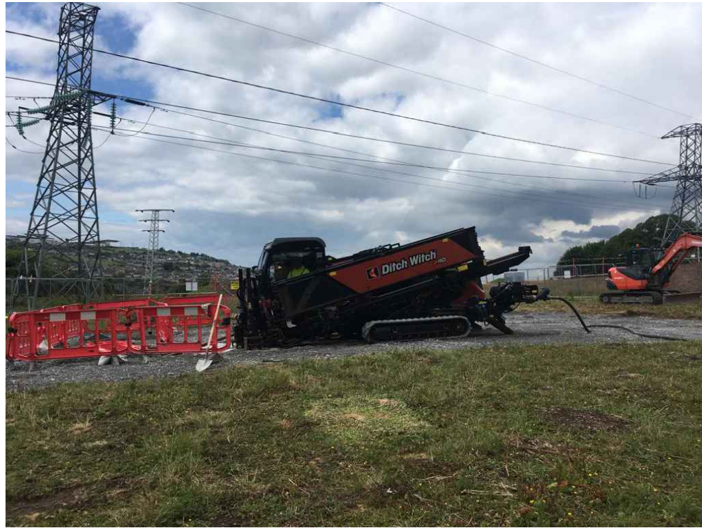
Image 1 : Typical Directional Drilling Rig
