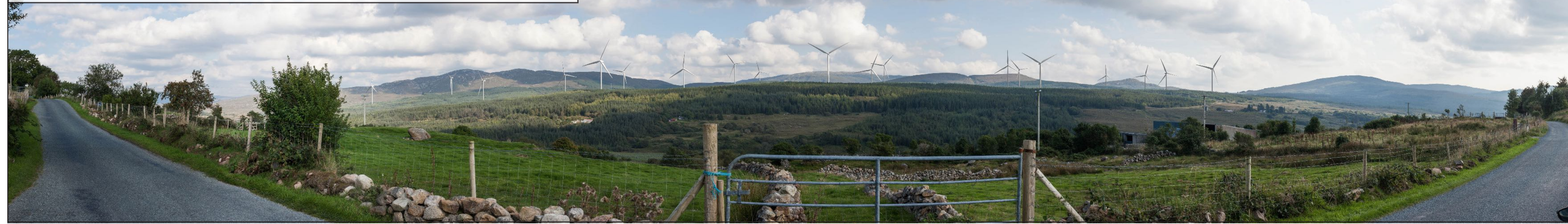
Alternative Scenario 2: Hub Height: 112m, Rotor Diameter: 164m, Tip Height: 194m.
