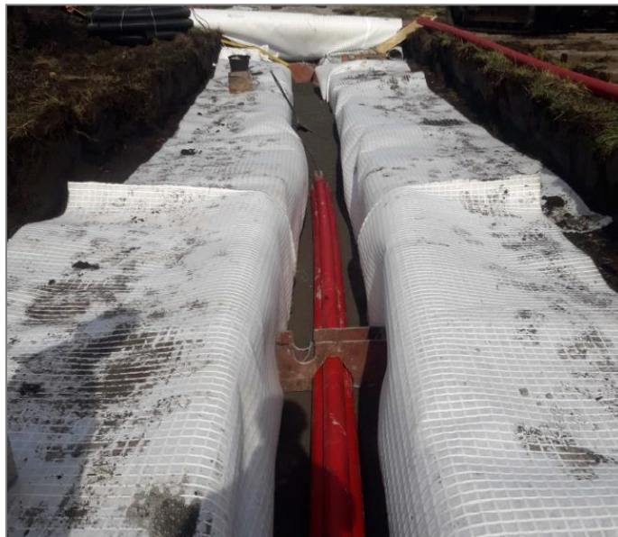
Figure 11 - Typical HV Underground Ducting Installation with geotextile membrane
