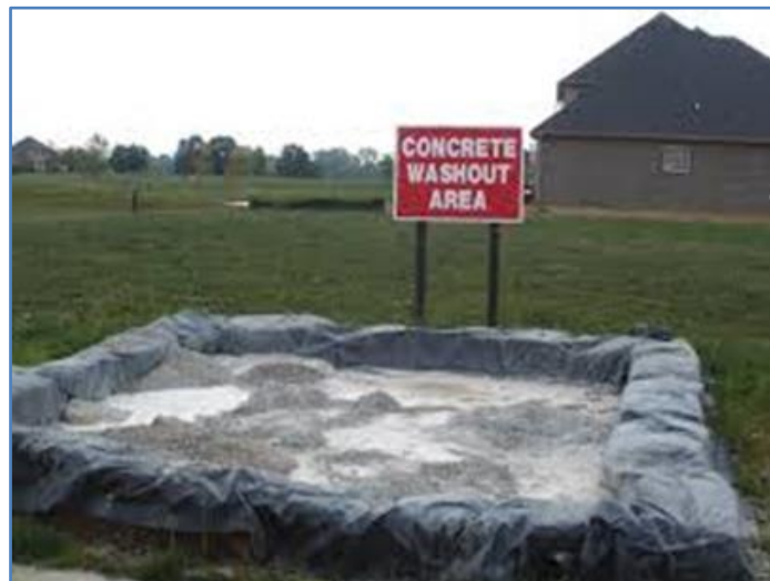
Photo 1 Example of a Concrete Washout Site
