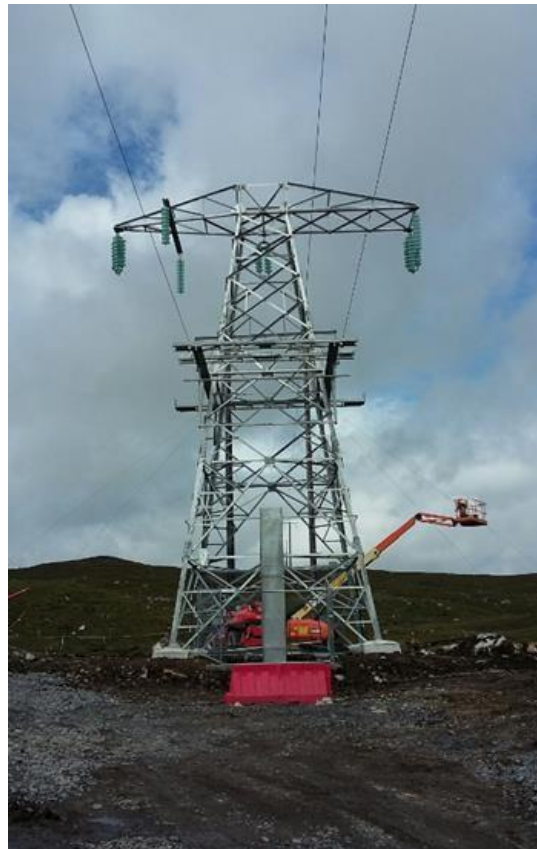
Figure 9 - Completed Line/Cable Interface Mas
