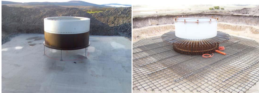
Plate 2-2: Levelled turbine tower “can” Plate 2-3: Steel reinforcement being added
