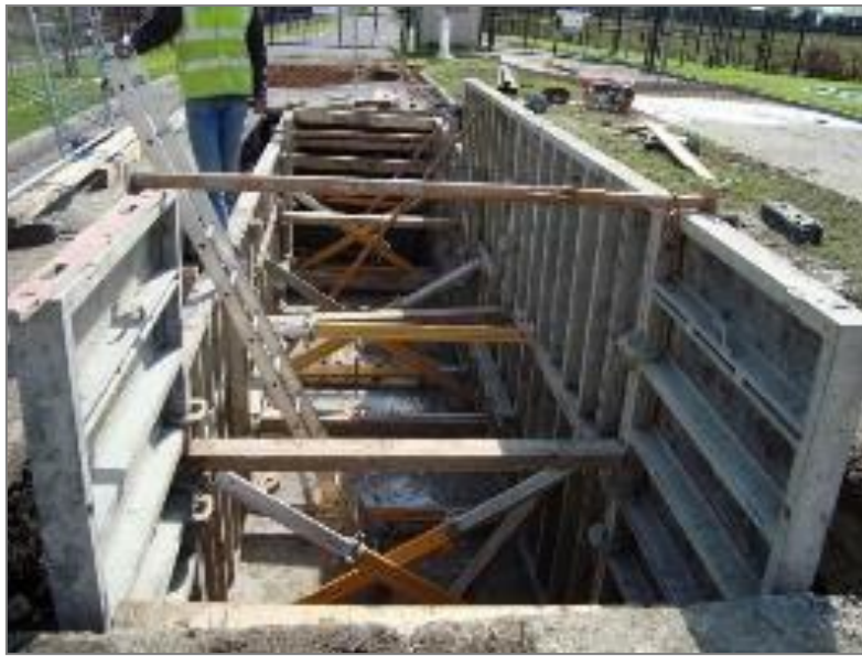
Figure 15 - Typical joint bay under construction (in-situ)
