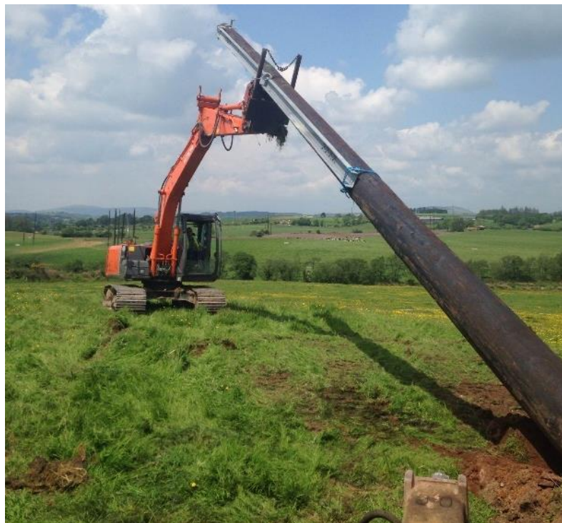
Figure 3 - Poleset removal with 13 Tonne excavator
