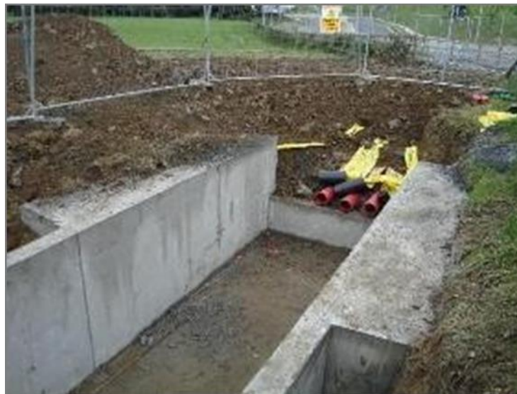
Figure 17 - Place pre-cast concrete sections on sand bedding.
