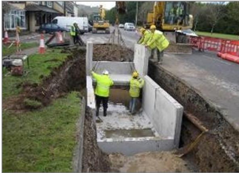
Figure 16 – Typical Joint Bay under construction (pre cast)
