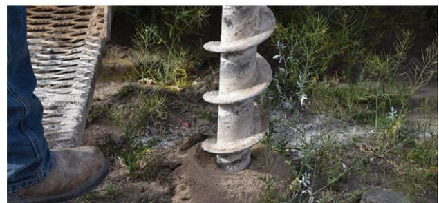
Image: Typical Auger drilling to obtain geotechnical ground samples
