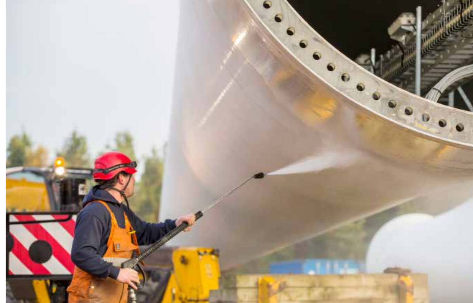
Turbine towers arrive in several parts and are assembled on site.
