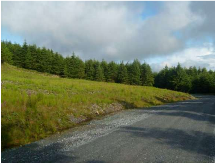
Photo 1 Good example of restored area filled with peat and sub soils
