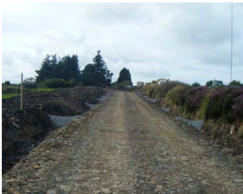
Figure 4.1 - Examples of Check Dams along Roadside Drainage Channels
