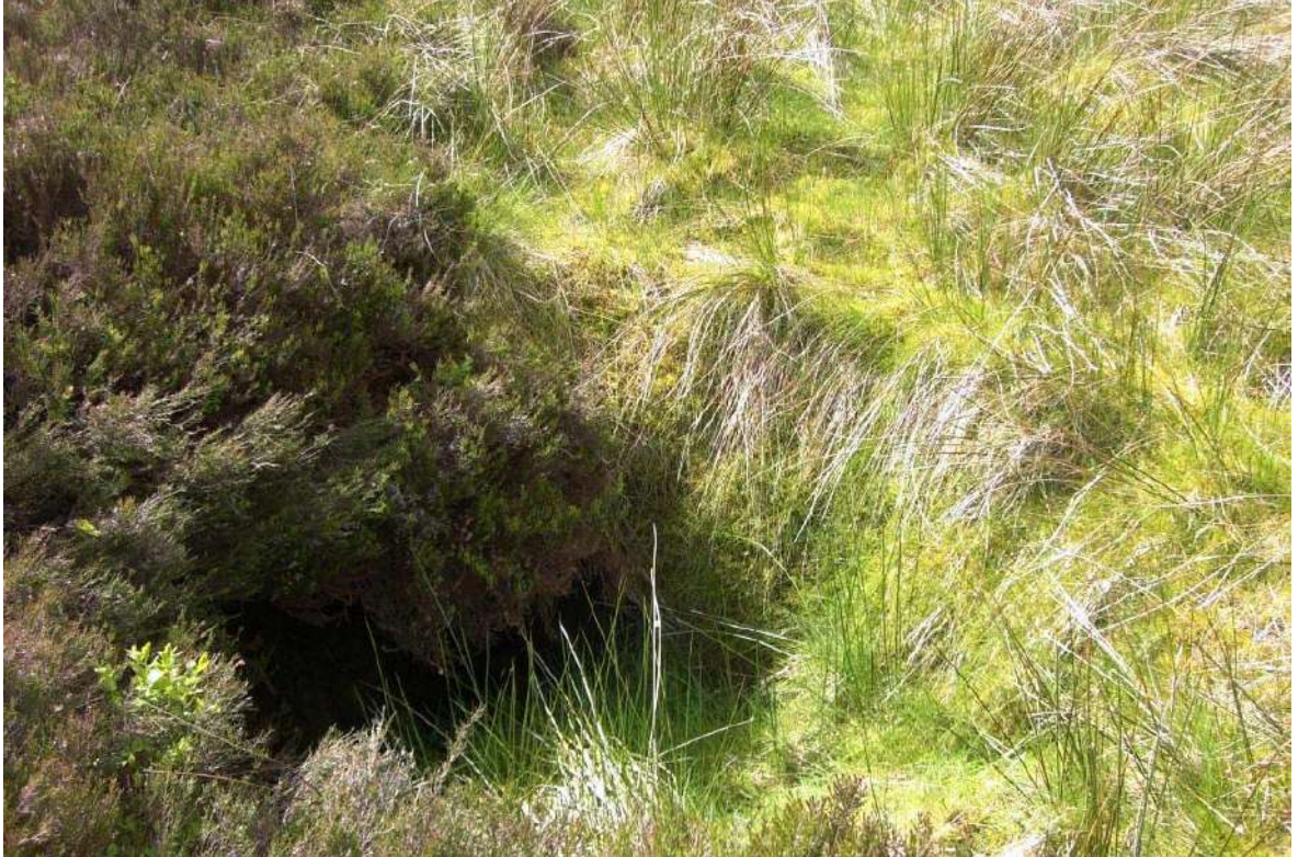
Figure 7 Collapsed Pipe Near E5 (view looking westwards)
