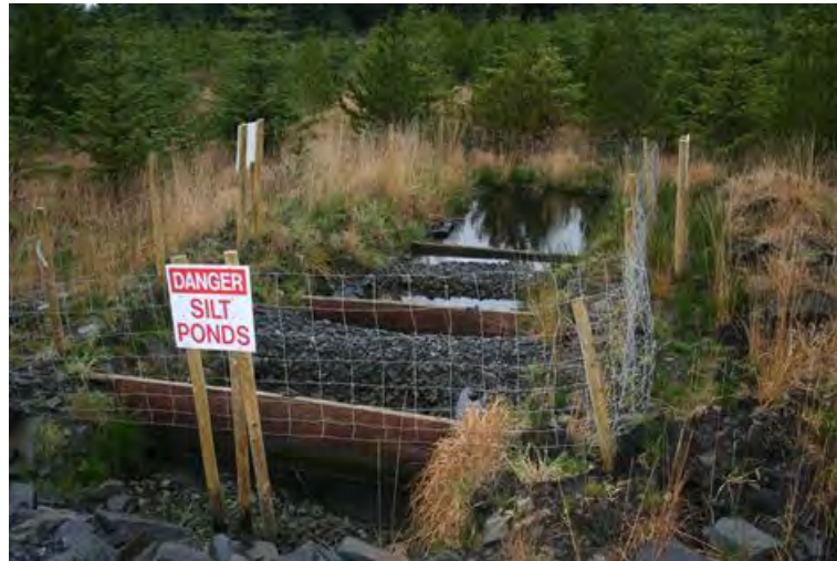
Figure 4.2 - Multi-tiered Sediment Basin with Stone Filter
