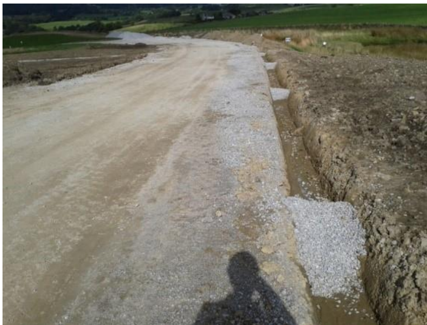
Plate 5.5: Check dam example
