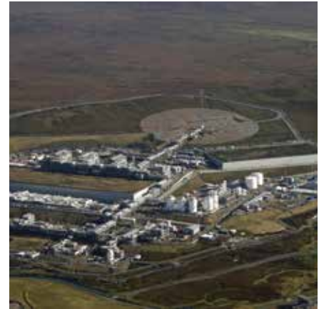
Shetland Gas Terminal
