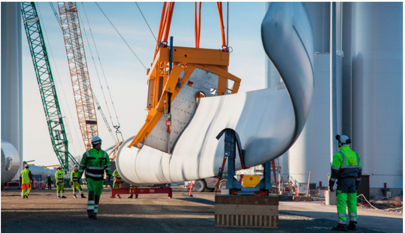
A blade for a wind turbine is ready to be installed at Anholt offshore wind farm
