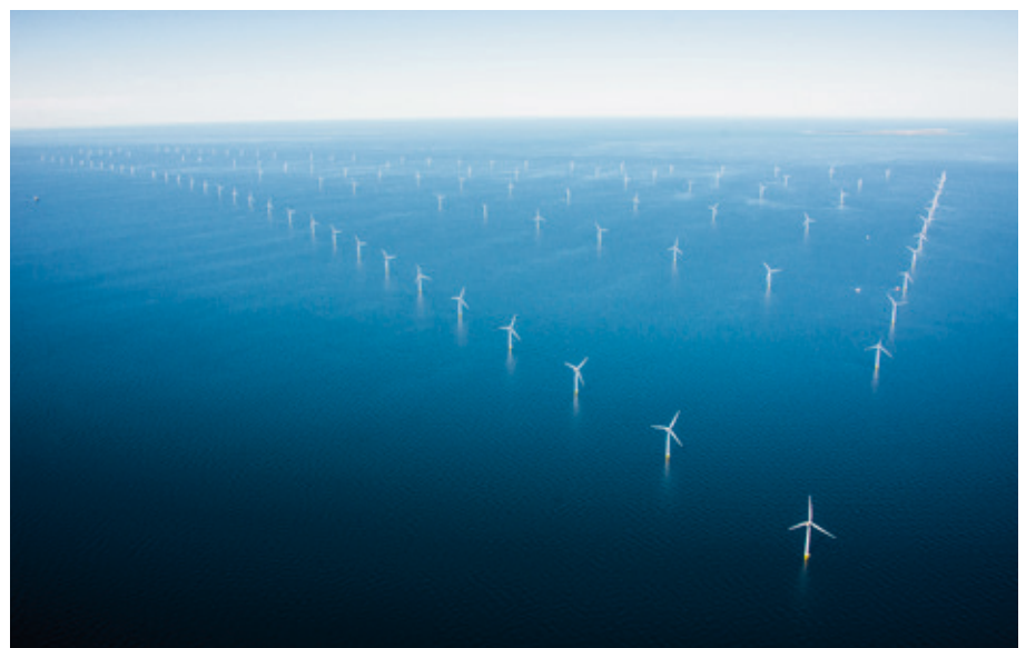
Anholt offshore wind farm
