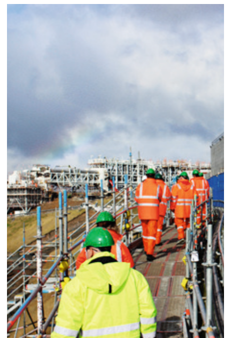
Activity at the Laggan-Tormore construction site
