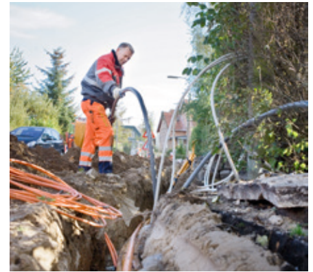
Cable laying north of Copenhagen in Denmark
