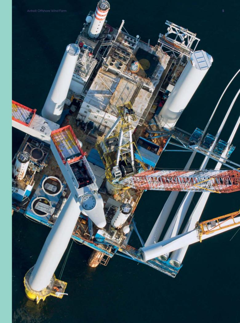
Installation lift at 82 metres. Each blade weighs 18 tonnes, and it takes calm weather and precision to lift the blades into place.
