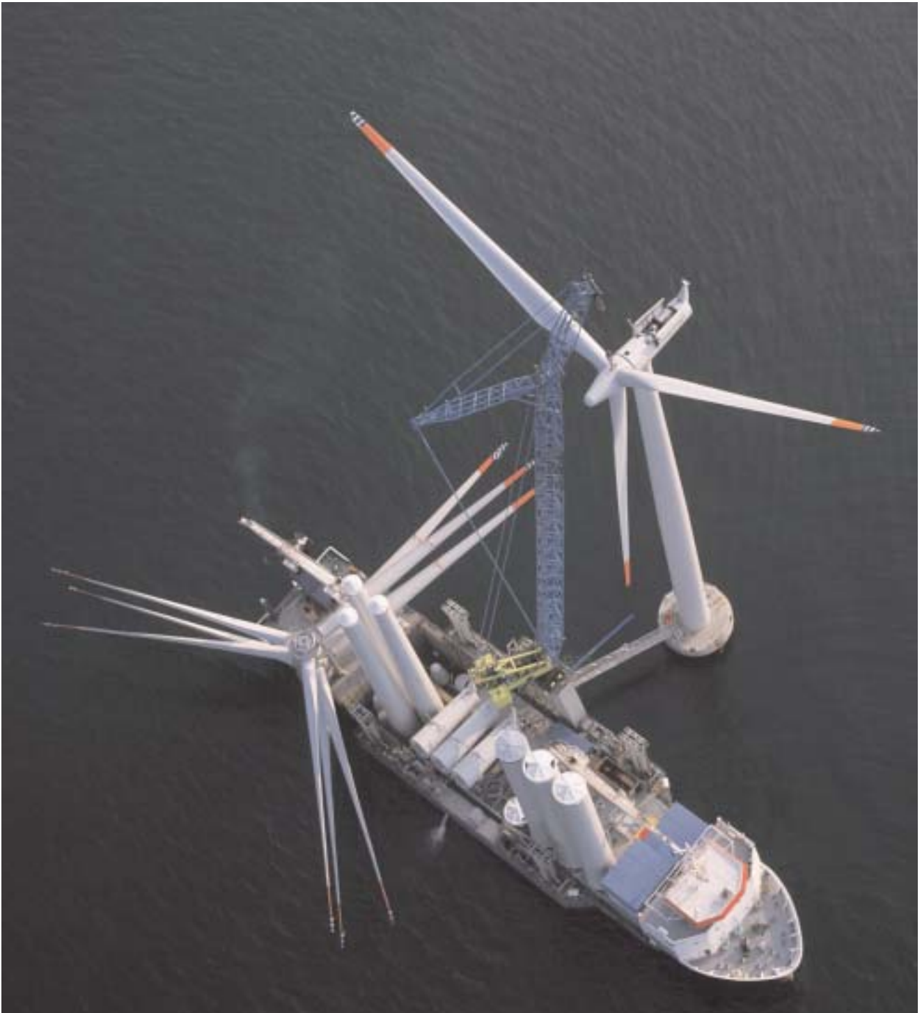
Erection of wind turbines, Nysted Offshore Wind Farm.
