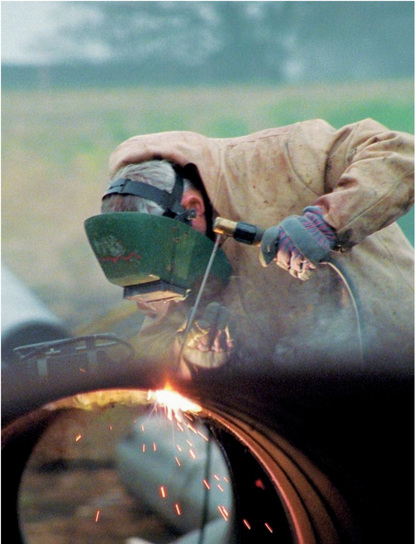
1980 – 1984: 800 kilometres of pipeline are laid for gas transmission through Denmark.
