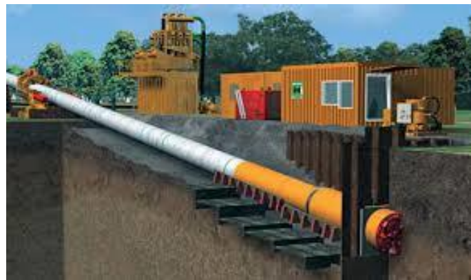
Figure 2.8. View of Direct Pipe technology [Source: http://www.indstt.com/pdf/HK_DirectPipe.pdf ]
