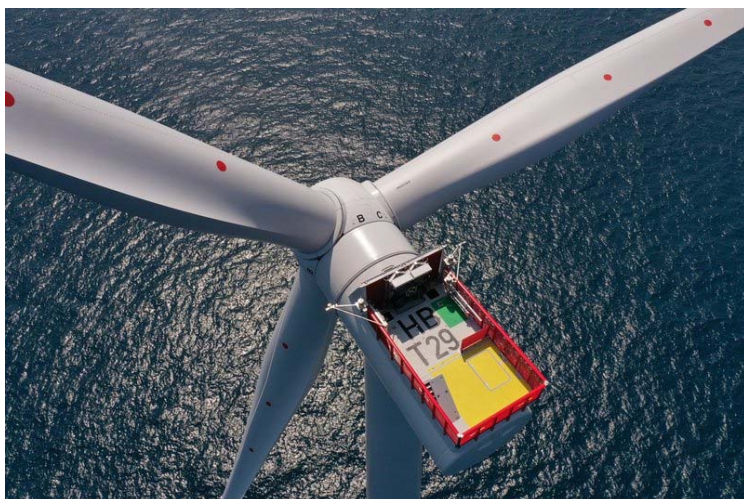
Installation of 1,000th offshore wind turbine at Hornsea 2, UK
