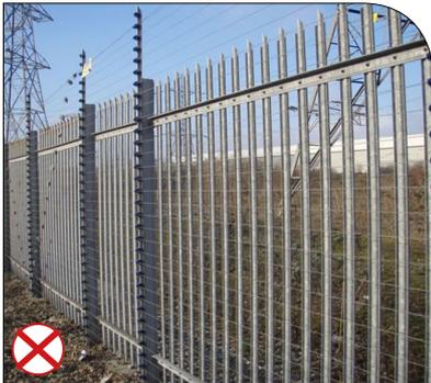
Galvanised steel security palisade fencing
