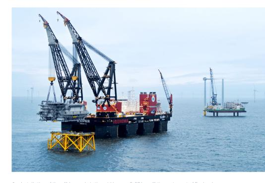
↑ Installation of the offshore substation at Hornsea 2, 89 km off the east coast of England.
